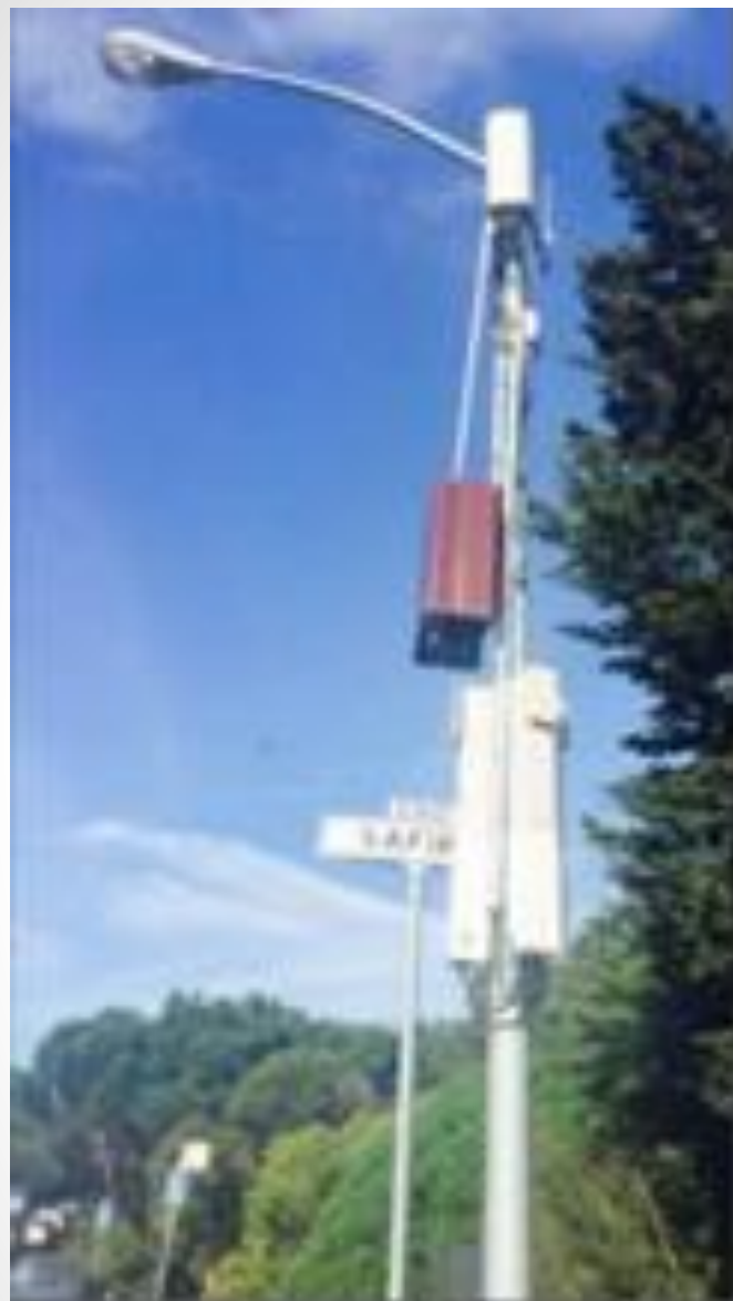
Actual Crown Castle Site. Modifications made w/o permits (whip antenna for Sprint, panel for Verizon)
