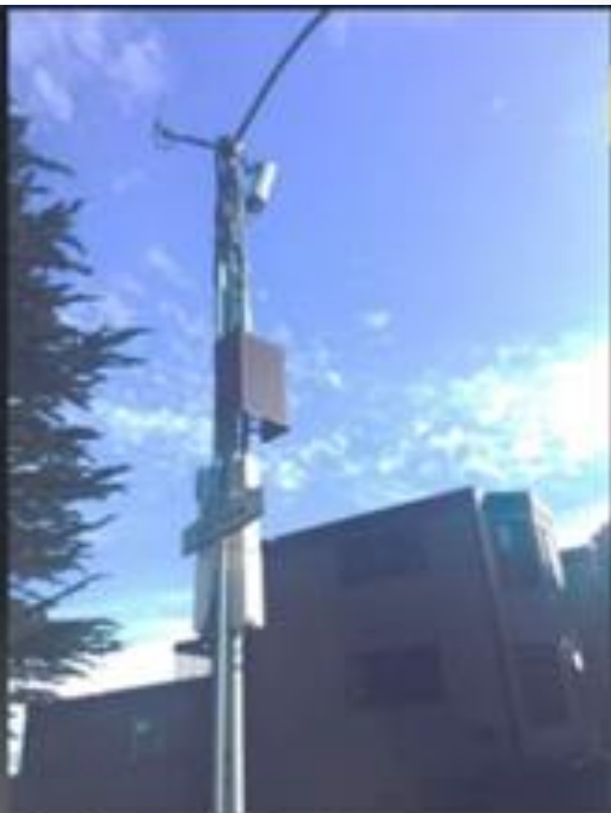
Actual Crown Castle Site. Modifications made w/o permits (whip antenna for Sprint, panel for Verizon)
